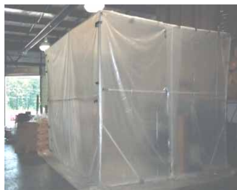
Photograph 2.4: AERC Ashland Facility - Containment Structure - Second Visit
